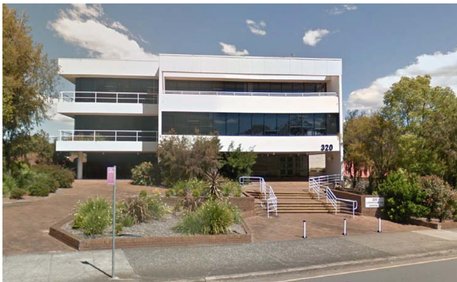
Figure 10- Existing commercial tower on Liverpool Road
